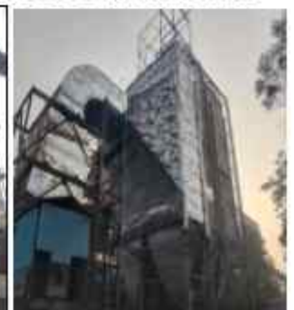
ESP of pellet plant
