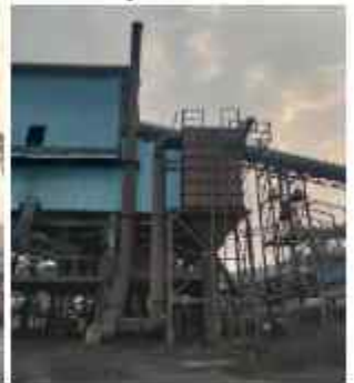
Coal Crusher Bag filter
