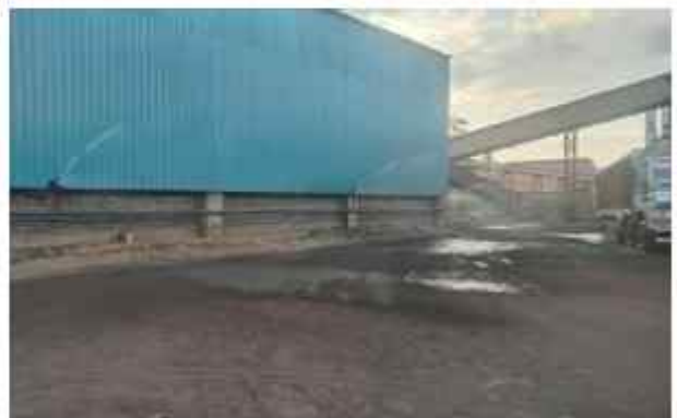
Fixed rotary type water sprinklers
